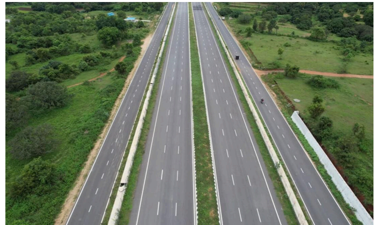
Six lane Bangalore - Nidigatta Section, 56.20 kms of NH-275 in State of Karnataka
